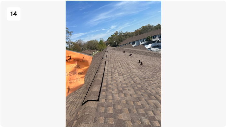
Project: MANHATTAN TOWNHOMES -BLDG 2 / 2402-5321019-01 Date: 2/28/2024, 1:38pm Creator: Maynor Perez
