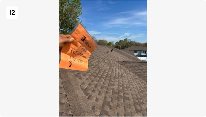
Project: MANHATTAN TOWNHOMES -BLDG 2 / 2402-5321019-01 Date: 2/28/2024, 1:37pm Creator: Maynor Perez
