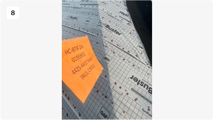
Project: MANHATTAN TOWNHOMES -BLDG 2 / 2402-5321019-01 Date: 2/26/2024, 6:09pm Creator: Maynor Perez
