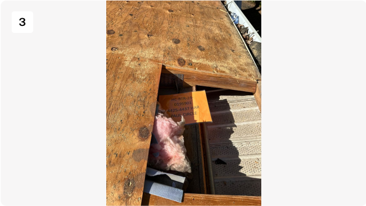
Project: MANHATTAN TOWNHOMES -BLDG 2 / 2402-5321019-01 Date: 2/26/2024, 11:43am Creator: Maynor Perez
